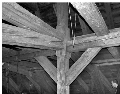
Figure 2.5.b. – Hardwood suspension bar – St. Michael church, Bamberg, Germany
